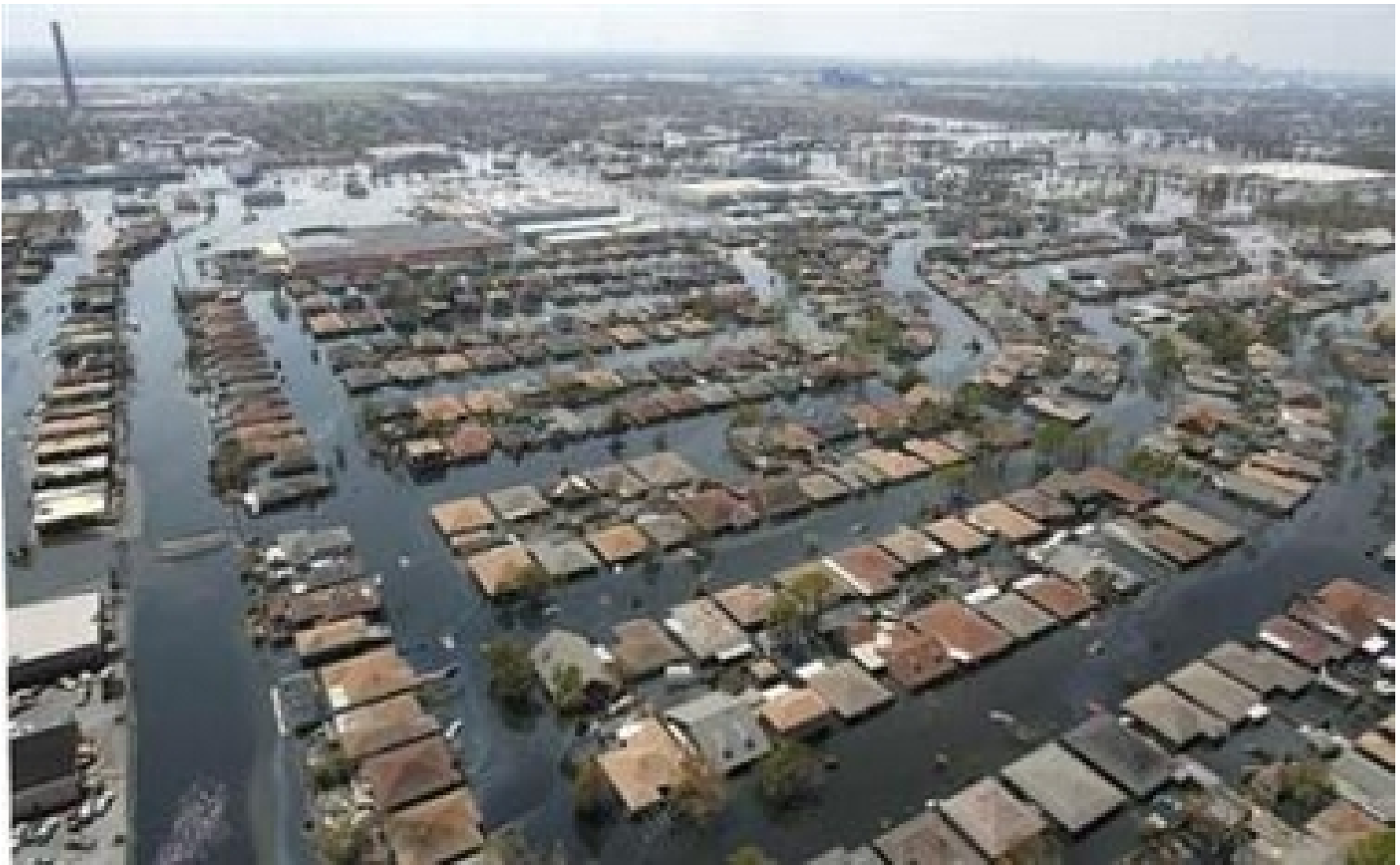
HURRICANE KATRINA FLOODING, NEW ORLEANS
